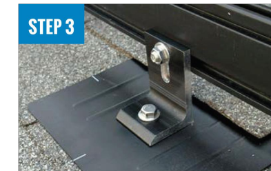
ATTACH L-FOOT TO RAIL
